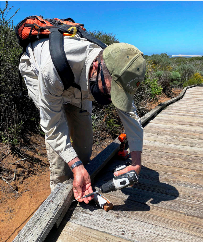
On April 27th, Rich Johnson wore a mask while repairing toe rails along the boardwalk. Photo by Prisila Johnson.
