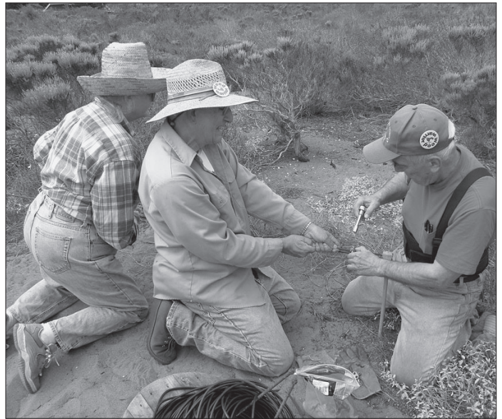
Weed Warrior Lannie Erickson (left) and Conservation Chair Pete Sarafian (center) pulled the symbolic fence cable tight while Ron Rasmussen fastened it to an anchor rod. Photo by Jean Wheeler
