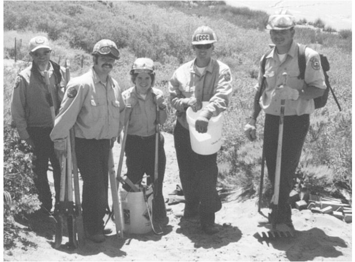
James "JT" Taylor (at left) and his CCC crew installed sand retention boxes at Bush Lupine Point to halt erosion on the sandy path behind them.
