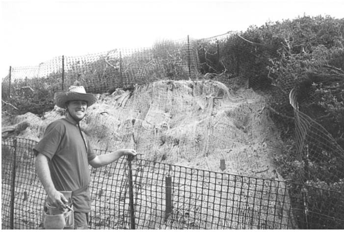
Josh Carmichael puts the finishing touches on his "jute taco," which will control erosion on the slope above Bush Lupine Point. Photo by Yolanda Waddell.
