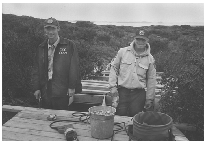
John Smith (left) and Mauricio, CCC Cadets, fasten boards in place on the last 200 feet of the boardwalk loop.
