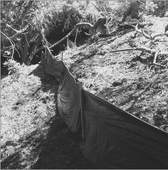
Removing a very heavy growth of the invasive Cape ivy from a grove at the west end of the Forest left a steep slope bare. Weed Warriors installed a silt fence to prevent erosion until native ground cover plants can grow in. Photo by Pete Sarafian.
