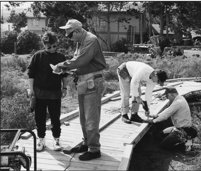
Below: Volunteers who pitched in and helped to install toe rails along the boardwalk included (l to r) Jan DiLeo, County Parks Planner, boardwalk architectural consultant Paul Wolff, neighbor Keith Wimer and Conservation Chair Pete Saraffian. Photos by Yolanda Waddell
