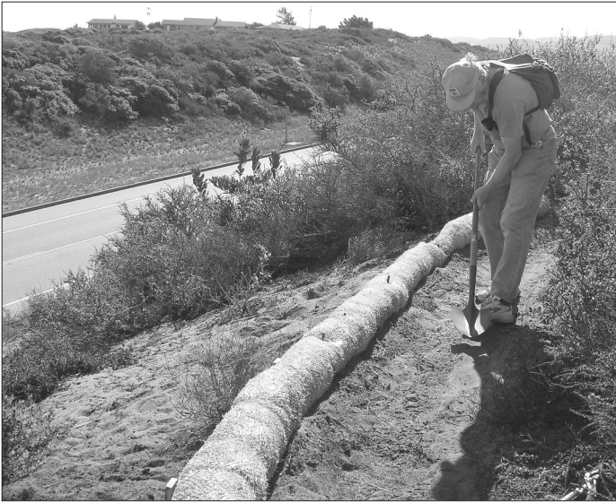
In November, the Weed Warriors replaced weather-beaten wattles at the top of the South Bay Boulevard embankment to control erosion of the loose sandy soil. Shown above is Steve Cake putting the finishing touches on a replacement wattle. Photo by Jean Wheeler.
